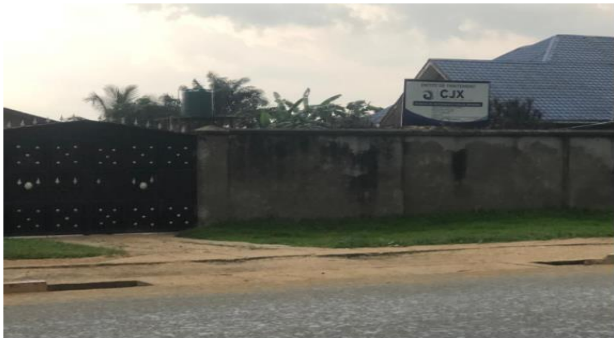
Figure N° 3 : Installation cjx Maniema
