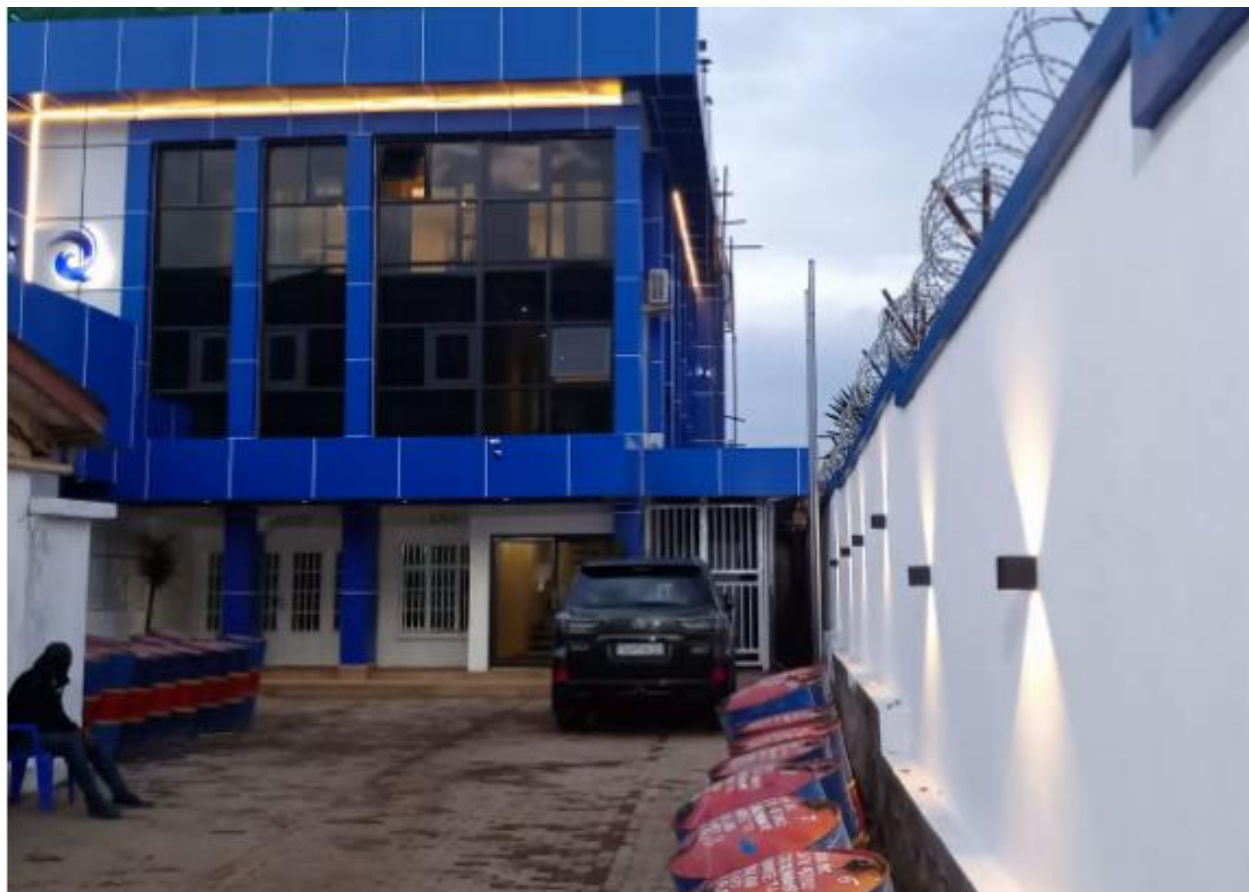
Figure N° 1 : Installation cjx Sud-Kivu
