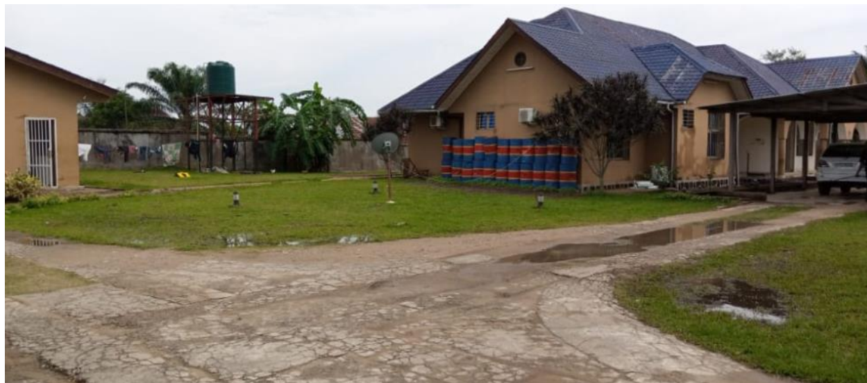
Figure N° 4 : Installation cjx Maniema
